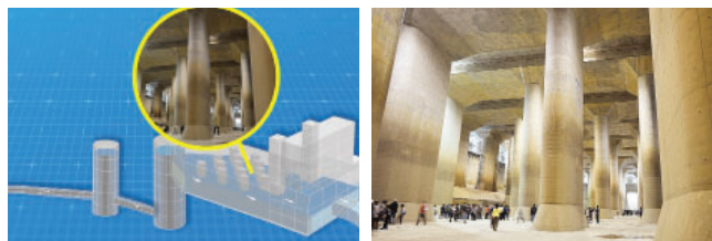
Tokyo's Underground Tunnel
