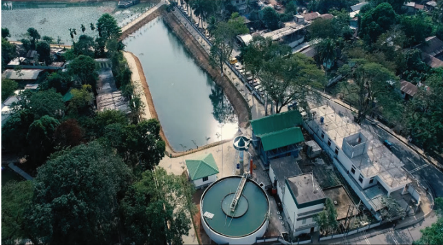
Rejuvenation of Jamuna Pond and Upgradation of Water Treatment Plant
