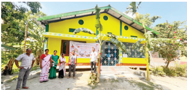
Griha Pravesh of a newly constructed PMAY(U) house
